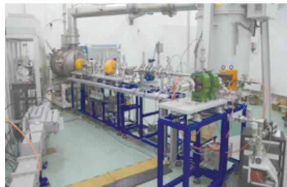
Fig.1 DC-SRF injector with beam line and 2K cold box
